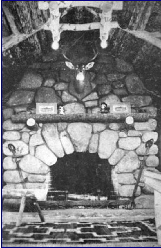
A fireplace and chimney breast of field stone, chosen with care and laid with more than average skill
