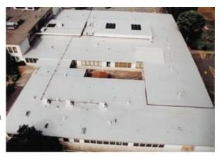
According to DOE, applying reflective aluminum flake to dark asphalt roofs is "an inexpensive, lightweight, [and] effective way to reduce the contribution that these types of roofs make to the air-conditioning power load."
