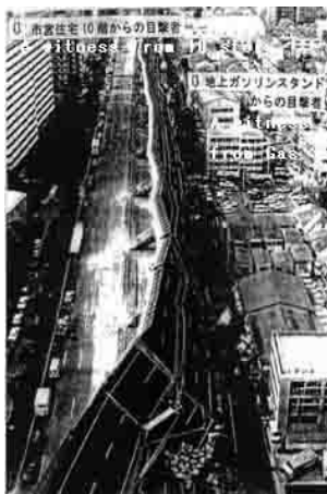
Photo.1 Overturning failure of Hanshin Highway and the location of watchers
