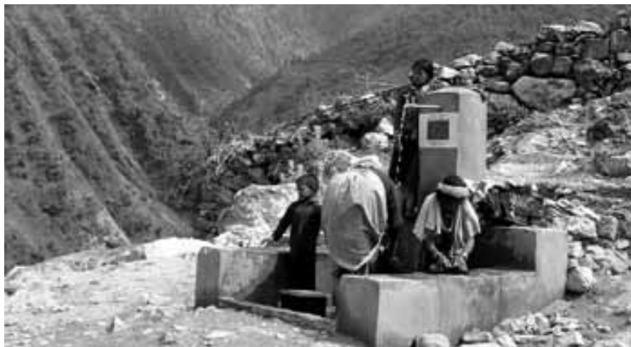
Tapstand gravity-fed water supply network in Basti village, Nepal
