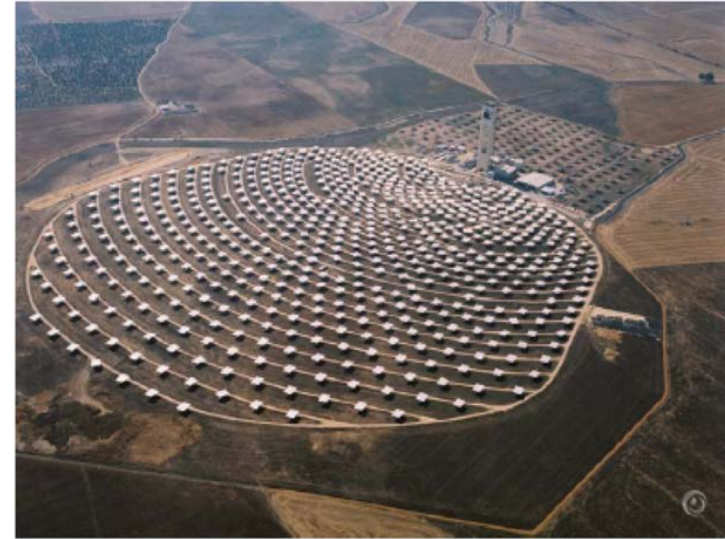
Aerial view of PS10 11MW solar plant
