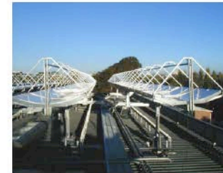
300m 2 Bruce Hall system under construction
