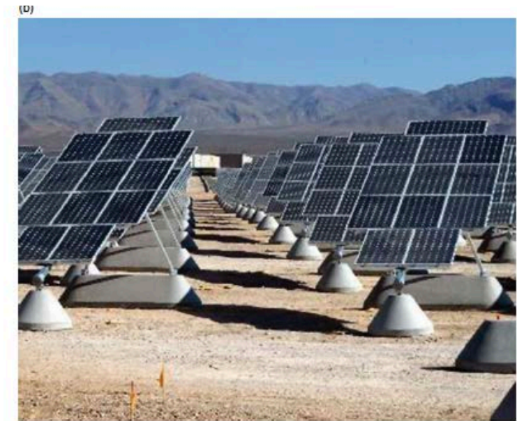
Figure 11.1.5 PV systems with (a) a single-axis horizontal tracker, and (b) a single-axis tilted tracker. Sources: (a) NEXTracker™ (2015); (b) Nellis AFB (2007)
