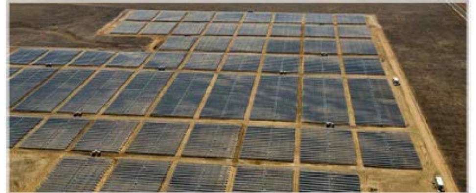
Figure 11.1.6 250 MWac ground-mounted system in California. Source: SunPower
