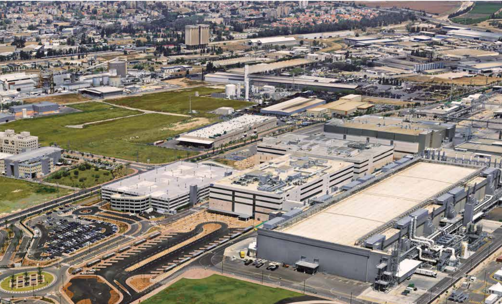
Photo courtesy Kiryat Gat Municipality
