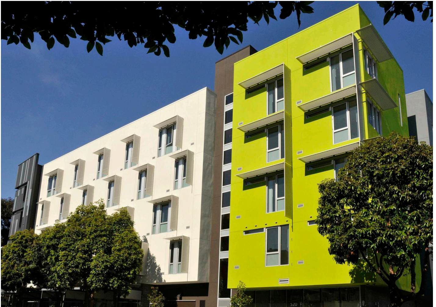
Richardson Apartments. David Baker + Partners
