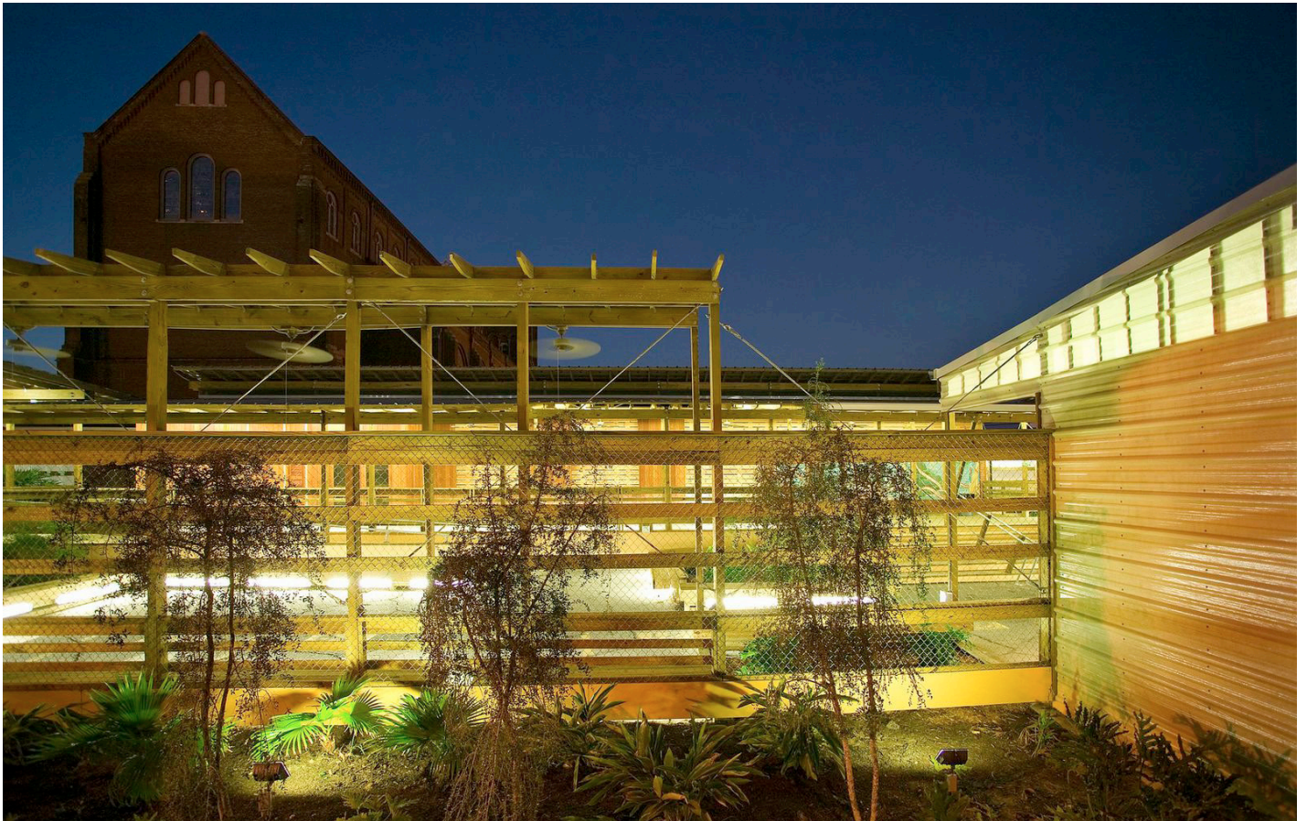
St Joseph Rebuild Center, New Orleans, Dan Pitera
