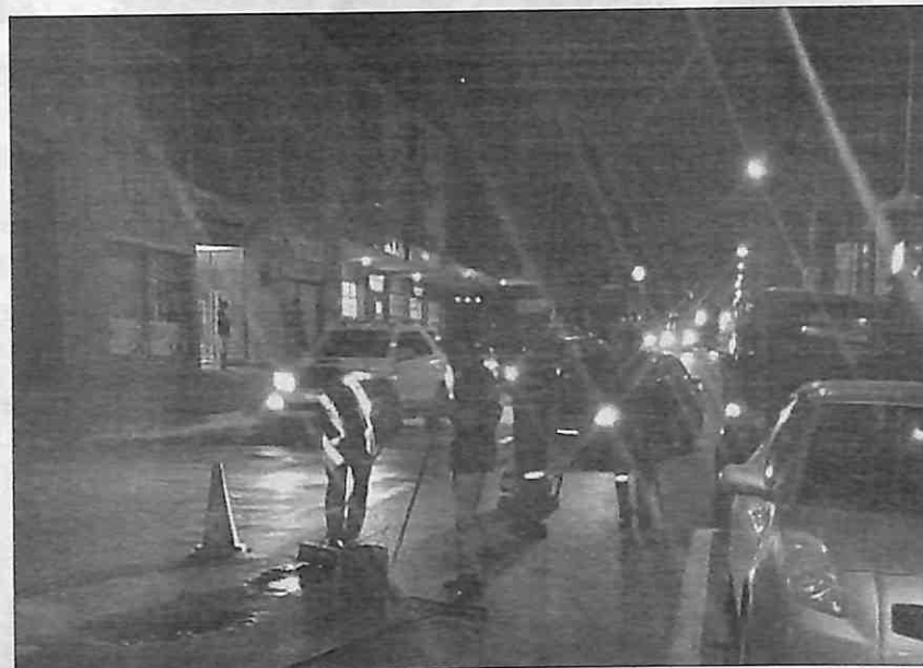
HIGH ACHIEVERS: Municipal Council of Manzini employees working at night to fix the roads damaged by the recent rains regardless of the festive break. They patched potholes using bitumen as well as re-gravelled and graded roads. (Pics: Nokuzola Thwala)
