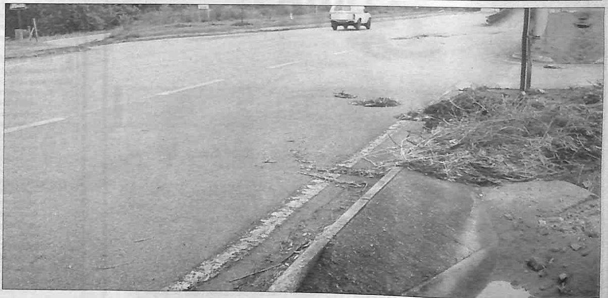
DANGER: The drainage system along the Malagwane Hill near Bahai School needs some special attention as it is now blocked and is forcing water into the road resulting in accidents. (Pic: Mduduzi Mngomezulu)
