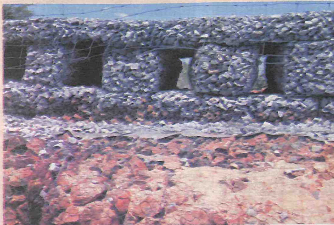
The installation of gabions protects further degradation of the soil.
