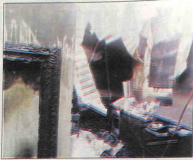
The heat of the inferno dislodged tiles from the walls in the kitchen.
