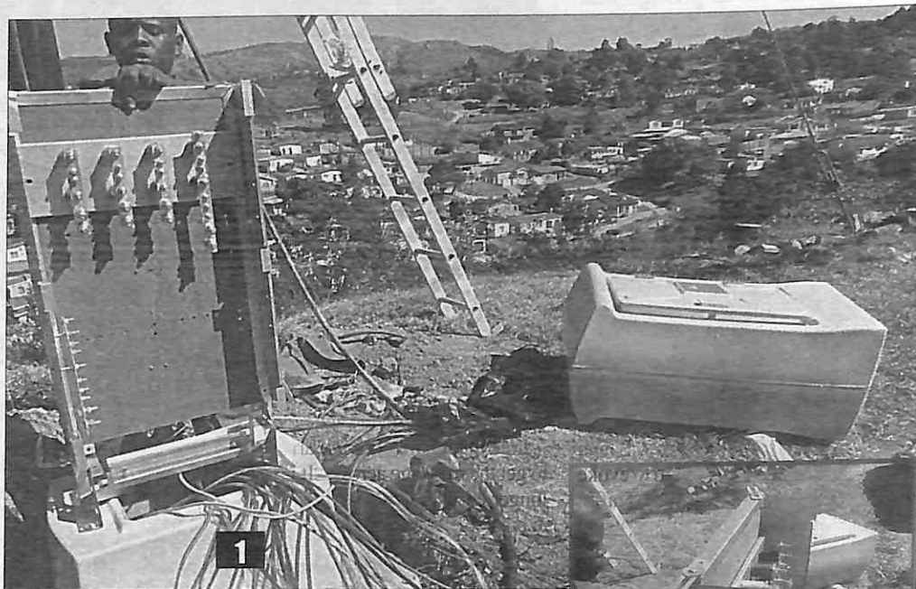
1. CONNECTING: An electrician found on the ground replacing the burnt kiosk.
