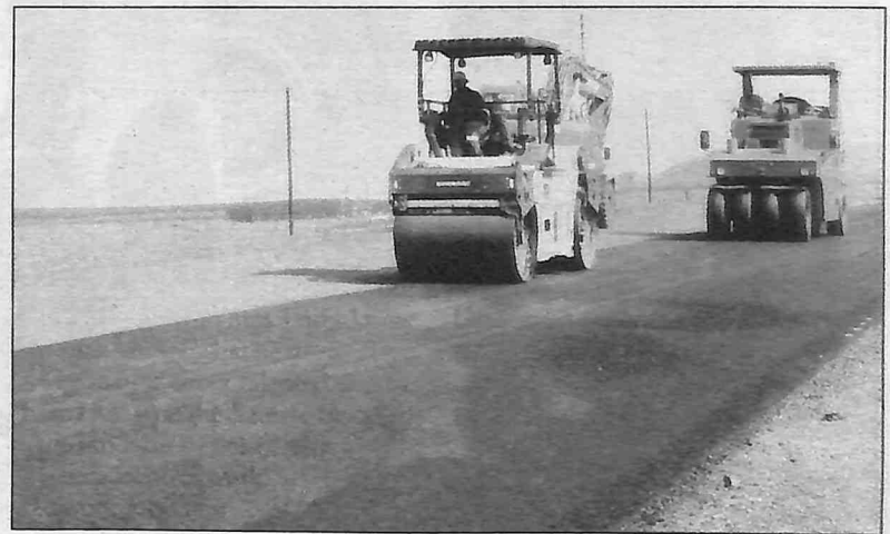
Machinery hardening the asphalt in the tarring of the 2km road from Gege towards Magubheleni.
