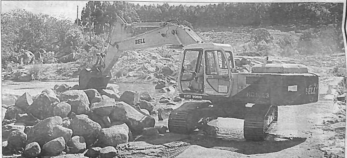
Another bridge at Mawelawela which is about 100metres away from the deadly one. Already, water is flowing above the low level bridge which is yet to be constructed.
