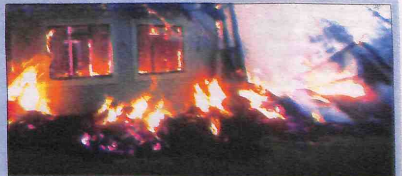
Nkonyeni gate house gatted by fire after lightning yesterday afternoon.
