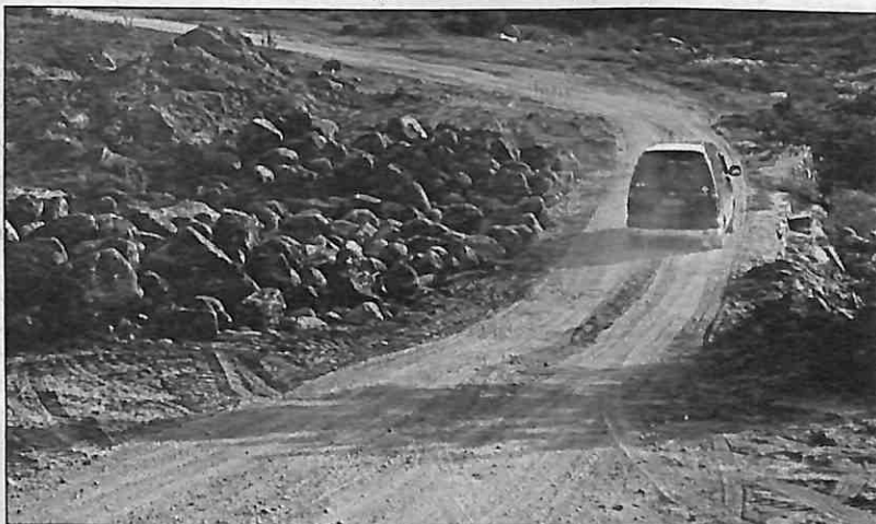
A vehicle crossing on the low level bridge which is 100 metres away from the 'killer' one. The ministry promised to reconstruct this bridge too, but nothing has been done on it so far.
