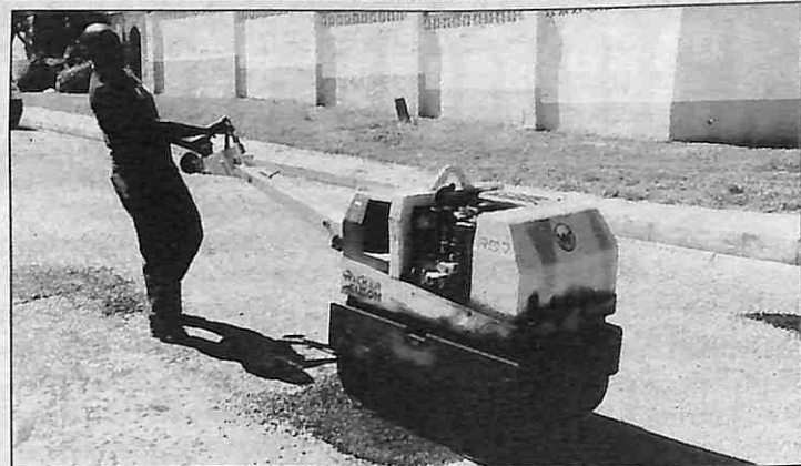
COATES VALLEY: An employee of the Municipal Council of Manzini busy patching potholes in Acacia road, Coates Valley, using a compactor.
