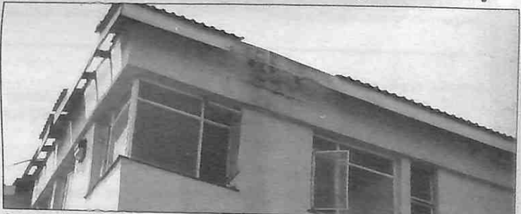
In some of the blocks, the roof has been blown away and remains unattended despite students' occupation in the blocks. The walls are also in a bad state and need a fresh coat of paint.
