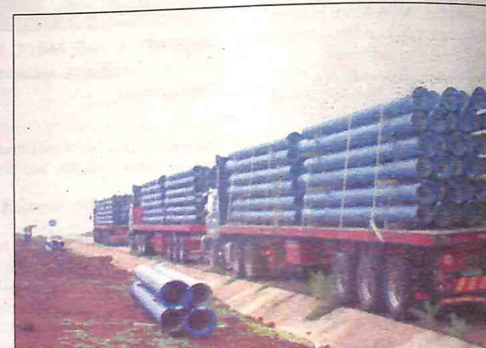
MORE PIPES: These are some of the ductile iron pipes that were being offloaded at the project site.
