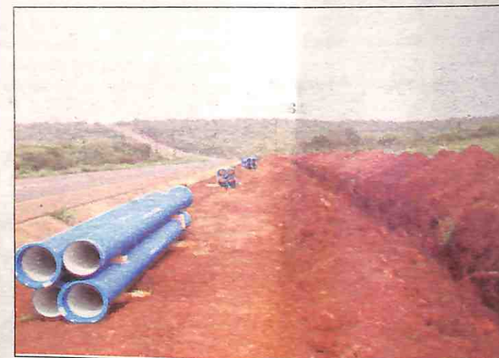
READY FOR BURIAL: These are some of the ductile iron pipes that will be connected for the project.
