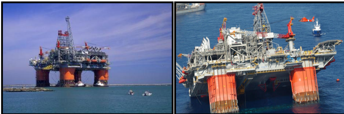
Figure 3.1 – BP Thunder Horse platform in the GOM severely listing and in danger of sinking.
