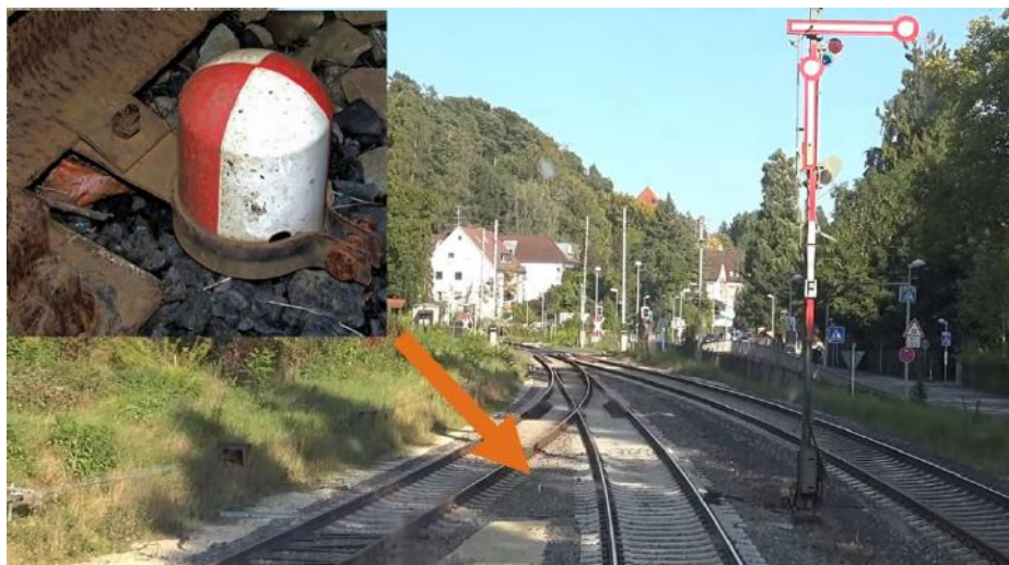
Figure 2: Example of a clearance point during recording. The recording was created with 60 frames per second and an approximate speed of 80 km/h. The entity is visible in the next 2 seconds.
