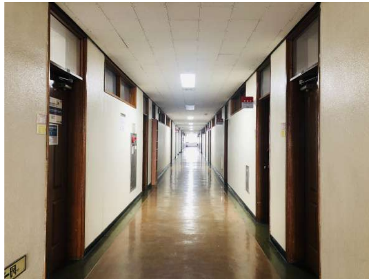
Figure 18. Real corridor environment on the 3rd floor of Kyungpook National University (KNU) IT-1 building.
