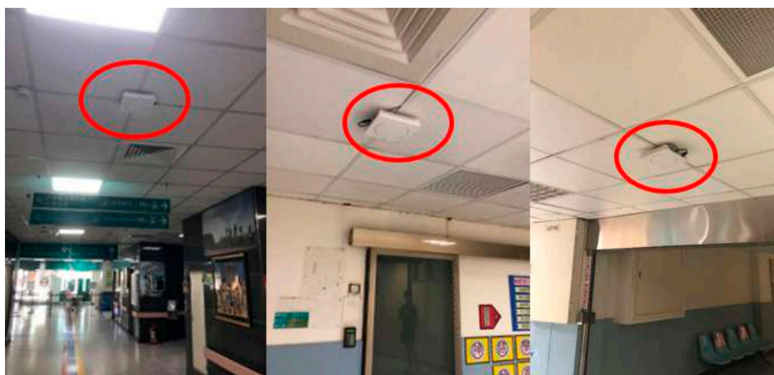
Figure 14. The installation of Lbeacons in the outpatient area of NTUH-Yunlin.
