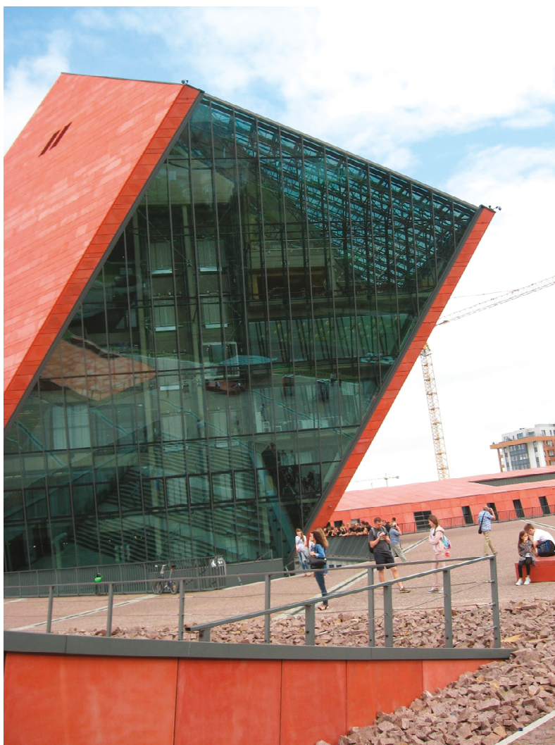
Figure 4. Gdańsk—Museum of the Second World War, main façade (photograph taken by J. Tymkiewicz).
