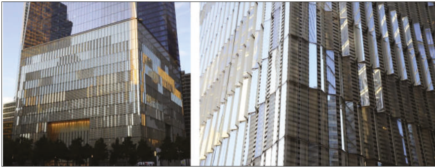
Figure 23. One World Trade Center: Reinforced concrete base with aluminum claddings and glass panels mounted in special profiles (photograph by authors).
