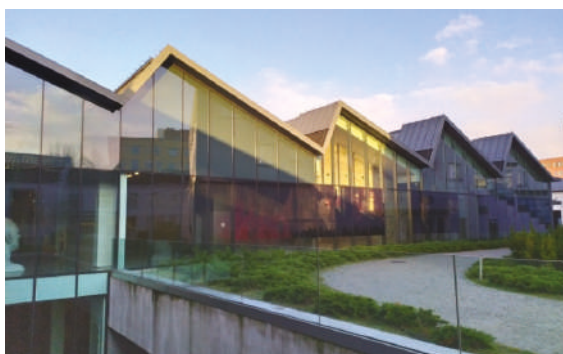
Figure 13. Museum of Contemporary Art in Kraków-MOCAK, designed by Claudio Nardi Architetture (Item 10, Figure 1) (photo by E. Latusek).
