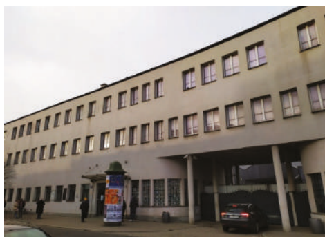
Figure 12. Museum-Oskar Schindler’s Enamel Factory in Cracow (Item 10, Figure 1) (photo by E. Latusek).
