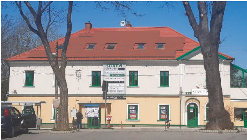
Figure 14. Harmonized color composition on the building's roof with the application of a new generation of color PV panels (computer simulation by P. Filipek).
