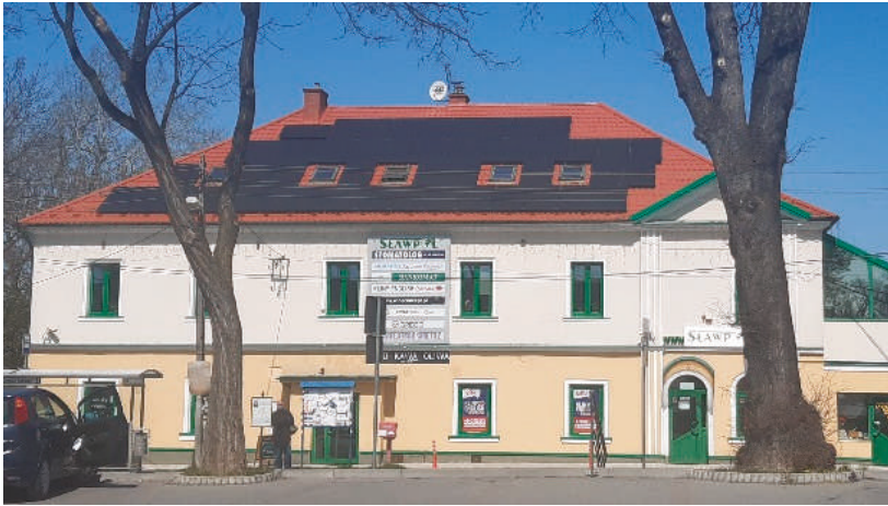
Figure 13. Disharmonious color composition on the building's roof covered with red ceramic tiles and monocrystalline PV panels (photo by W. Celadyn).
