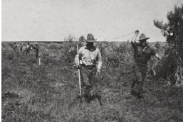
Surveying team measuring a baseline distance with a metal (Invar) tape. (Hodgson, 1916).
